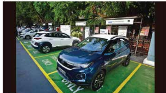
The first set of NHEV's charging stations -- totalling eight with two each in the north, south, east, and west zones -- will be operational by March 2023.
